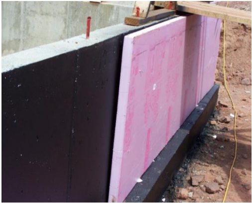
Exterior insulation R-10 continuous
