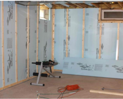
Interior insulation R-15 continuous
